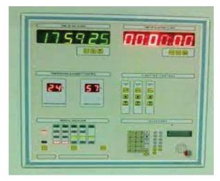
All the control for the modular operation theatre are located on a membrane base control panel flush mounted in the theatre wall panel. A remote electrical distribution board is provide to allow access the panel for repairing without any problem access to the theatre Each Control panel contains:
